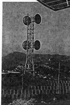
Telecommunications system in Greece
